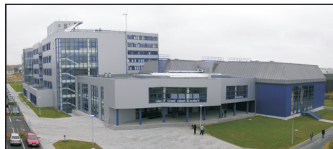
Faculty of Electrical Engineering building the venue of the conference Applied Electronics
